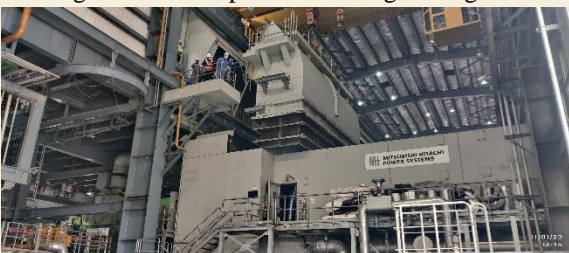
Figure: GT Air Inlet Duct installation
