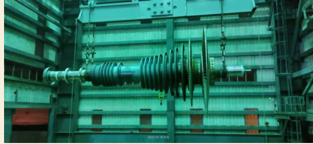
Figure: Steam Turbine Rotor Lifting work
