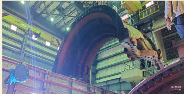
Figure: GT Turbine Casing Lifting Work
