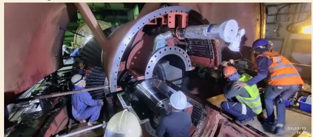
Figure: GT Exhaust Casing Installation Work
