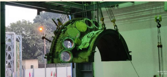
Figure: GT Comp-Comb Casing Lifting Work
