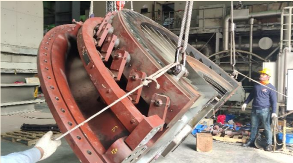
Figure: GT Inlet Casing Turning Over Work
