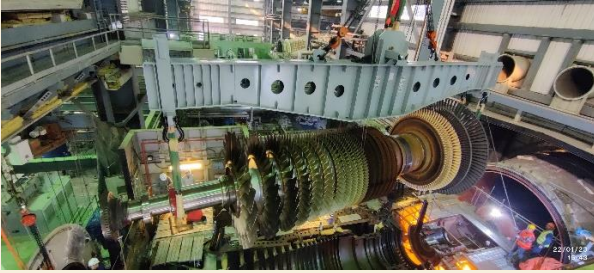
Figure: Gas Turbine Rotor Lifting work
