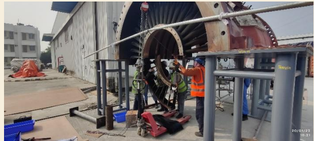
Figure: Diaphragms removal from compressor casing
