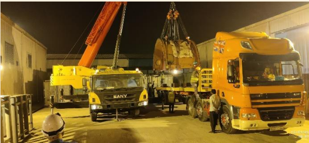
Figure: GT Turbine casing placing at laydown area
