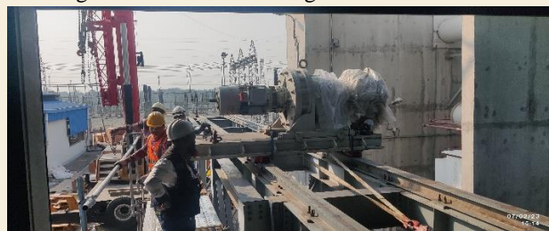
Figure: GT Turning Gear Transportation Work
