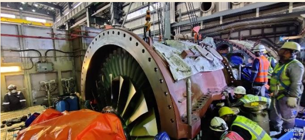
Figure: GT Compressor Casing Installation Work
