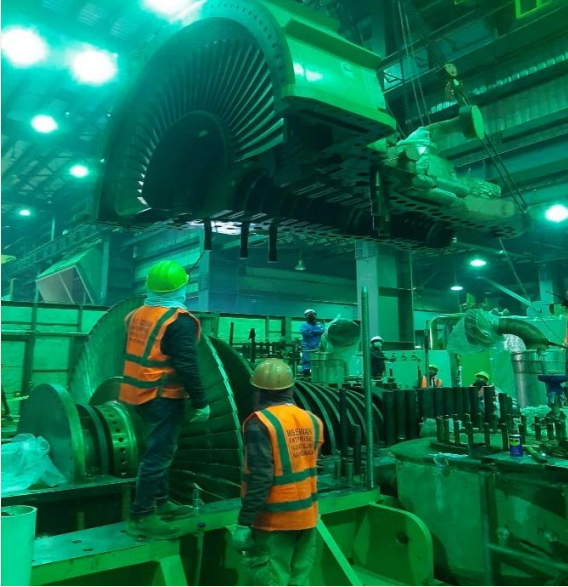
Figure: ST HIP casing lifting work
