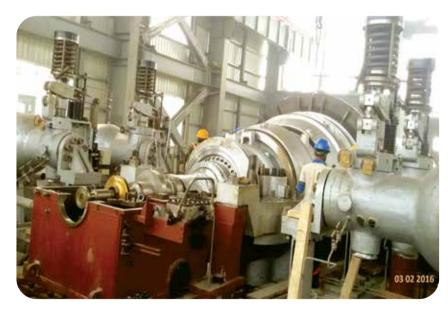
Erection of Turbine of Upgradation of Khulna 150 MW to 225 MW CCPP Project
