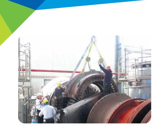
Removing of Turbine's Upper Casing during HGPI Work at Sirajganj 225 MW CCPP
