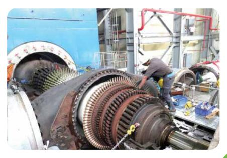
Removing of Turbine's Old Blades during HGPI Work at Sirajganj 225 MW CCPP
