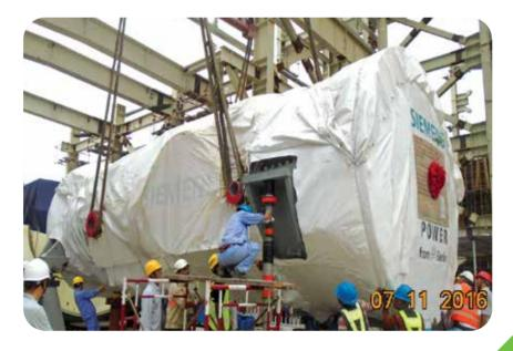
Placing of Gas Turbine for Sirajganj 225 MW CCPP Project (2nd Unit)
