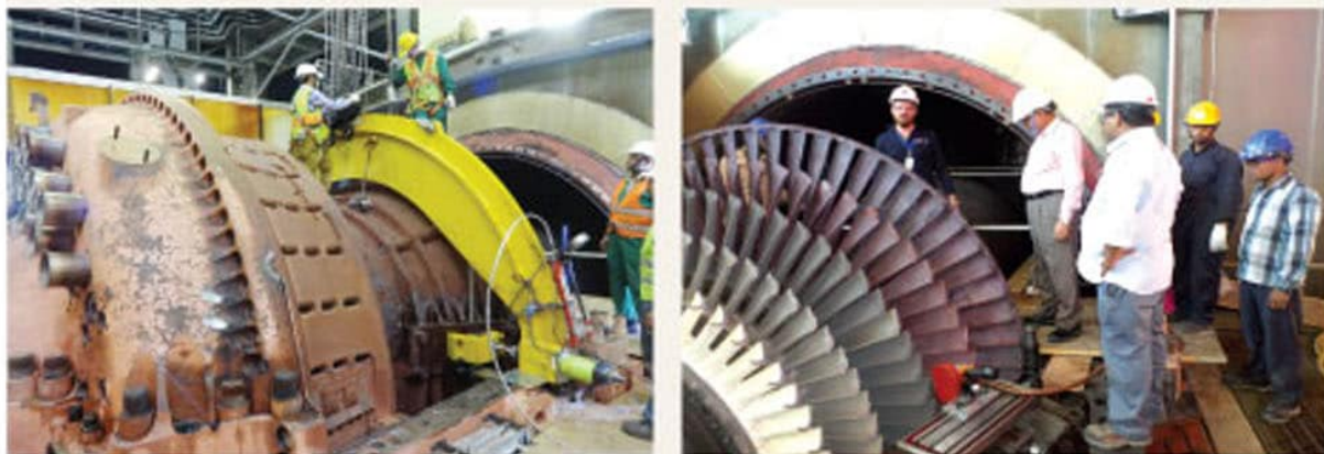
C1 Inspection of Khulna 150 MW PPP
