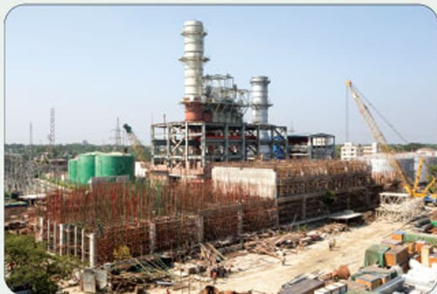
EPC Work Upgradation of Khulna 150 MW PPP to 225 MW CCPP Project
