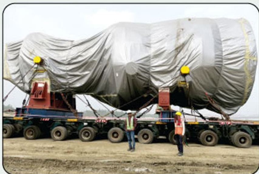
Movement of Gas Turbine Bheramara CCPP (360 MW) Development Project
