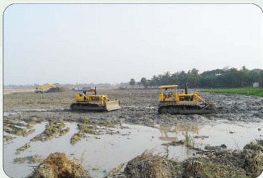
Development work of Payra 1320 MW TPP Project
