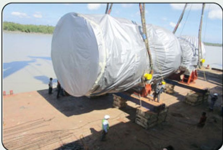
Gas Turbine unloading to the Barge Bheramara CCPP (360 MW) Development Project
