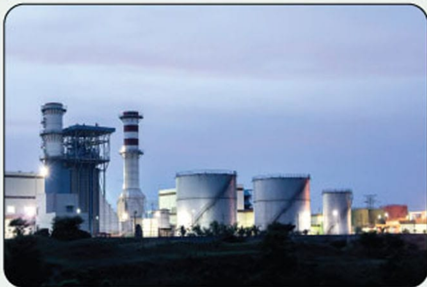
Sirajganj 225 MW Combined Cycle Power Plant
