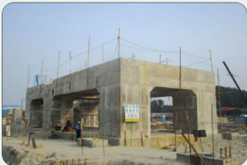
STG Foundation Bheramara CCPP (360 MW) Development Project
