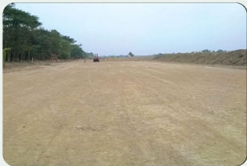
Embankment work of Payra 1320 MW TPP Project
