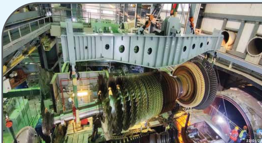
1st Major Overhaul Inspection of Bheramara 410 MW CCPP (10 Jan 2023 to 18 Feb 2023)
