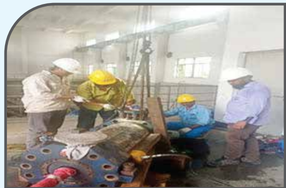
Major Overhaul of Boiler Feed-Water Pump (BFP) of Sirajganj 225 MW CCPP Unit-1 (27 Sep 2022 to 15 Oct 2022)
