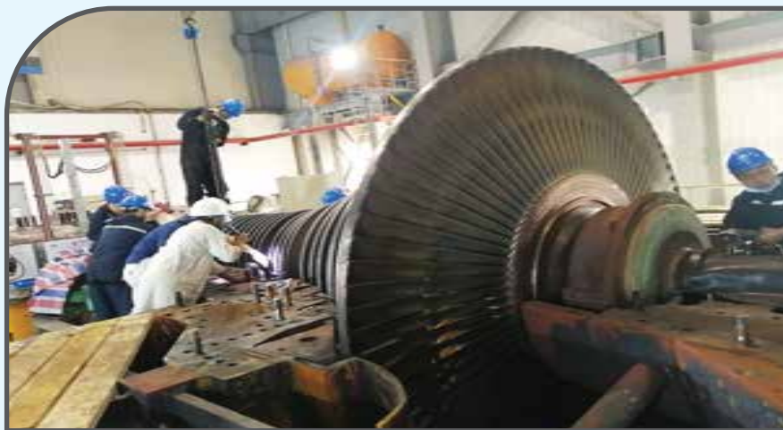
1st Major Inspection (MI) of Steam turbine
