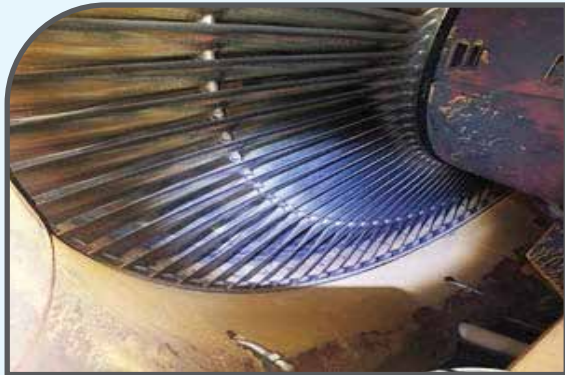
Last stage inspection of ST
