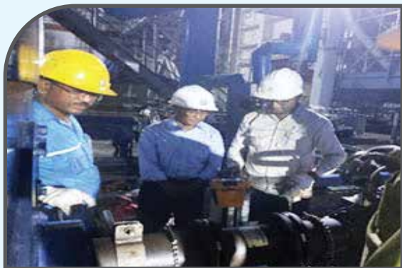
Major Overhaul of Boiler Feed-Water Pump (BFP) of Sirajganj 225 MW CCPP Unit-1 (27 Sep 2022 to 15 Oct 2022)
