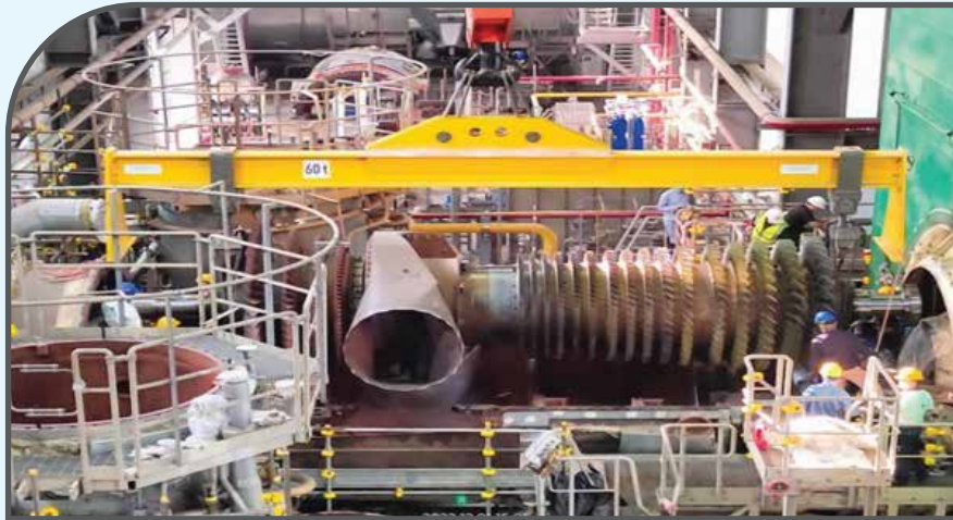
GT Compressor disassembly
