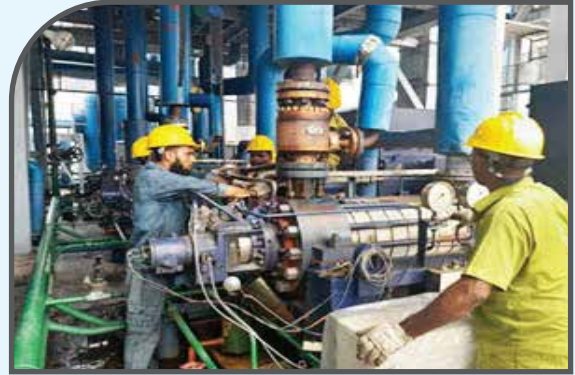
ARC valve replacement of BFP (A & B)
